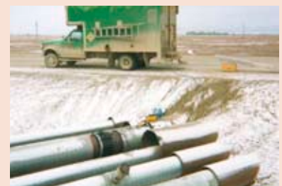
Road crossing on the North Slope
