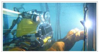
Underwater welding being carried out. Courtesy of Hydroweld UK.
