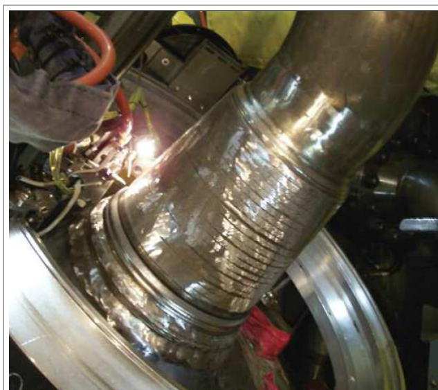
Full strength weld overlay applied at AmerenUE's Callaway nuclear power plant. Courtesy of the American Nuclear Society.
