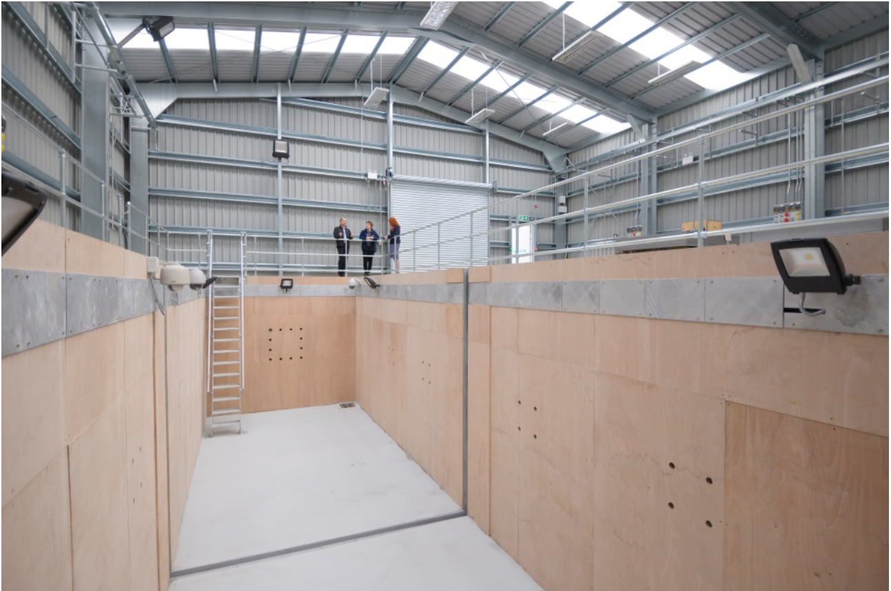
TWI pressure pit facility to be used for the large scale pressurised tests on a representative vessel
