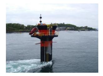
The system will be validated by installing it on an inservice tidal stream generator developed by one of the SMEs who will also be an end user of the proposed REMO technology.
